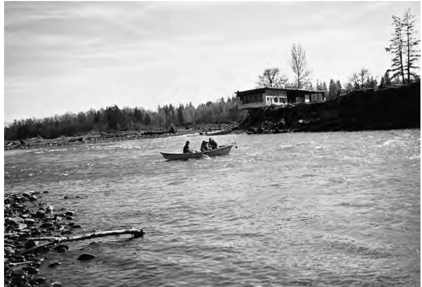
Figure 17. Building undercut by bank erosion as the Clackamas River flows through a captured gravel pit near Barton, Oregon. (Photograph by the author, April 1996.)
