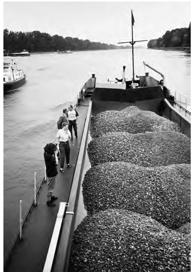
Figure 5. Barge artificially feeding gravel into the River Rhine downstream of the Barrage Iffezheim. (Photograph by author, June 1994.)
